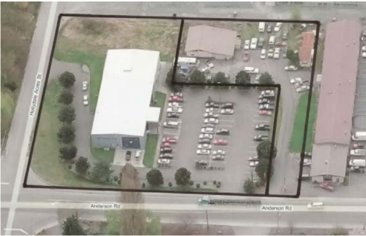
An aerial picture of the JATC Training Center Expansion.
